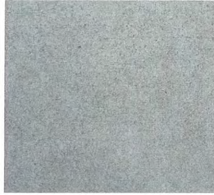
Production Concrete Paving - Natural Gray with Light Top-cast Finish & Saw-cut Joints.
