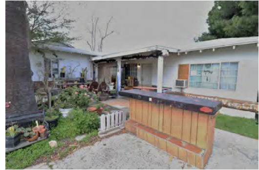
Figure 3: South elevation, east end, view north (LSA 2021)
