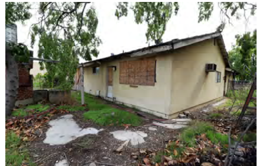
Figure 5: North (left) and west (right) elevation, view southeast (LSA 2021)
