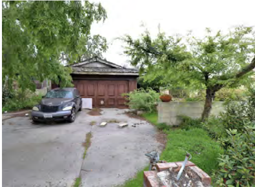
Figure 2: South elevation, view north (LSA 2021)
