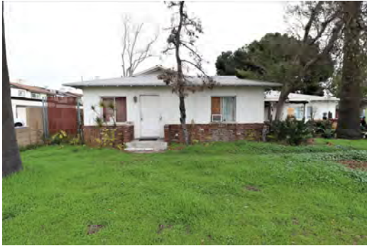
Figure 2: South elevation, western projection, view north (LSA 2021)
