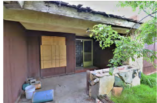
Figure 3: Main entrance, view north (LSA 2021)
