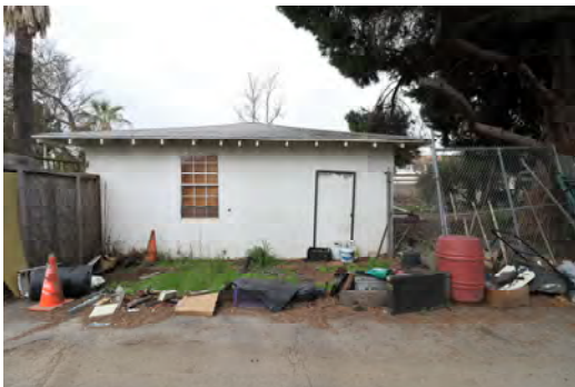
Figure 4: East elevation, view west (LSA 2021)
