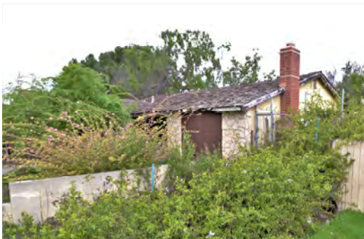
Figure 4: South (left) and east elevation (right), view northwest (LSA 2021)
