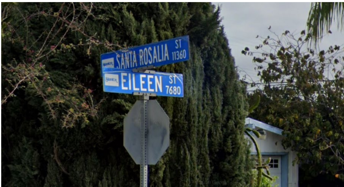
Note: Peeling of the anti-graffiti coating can be seen in these photos.
