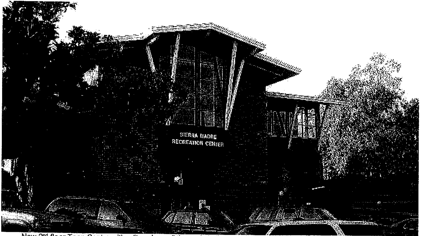
New 2 nd floor Teen Center with a "tree house" theme is built over existing 1 st floor Community Center
